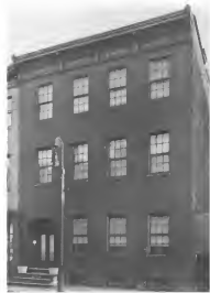
The Craig house, 913 East Pratt Street, in the early 20th century. The house was originally only two and a half stories high with a sloped roof and attic dormers; the third story and new cornice were added about 1875. The building was demolished in 1995.
